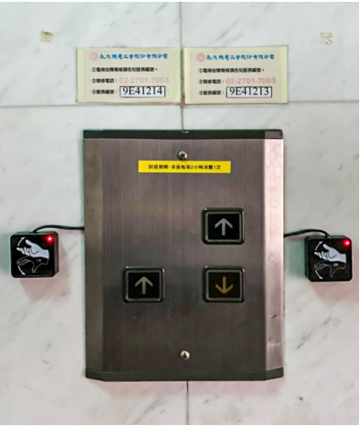
Hand gesture sensors are installed on elevator panels to reduce contact.
