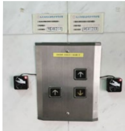
▲ Hand gesture sensors are installed on elevator panels to reduce contact
